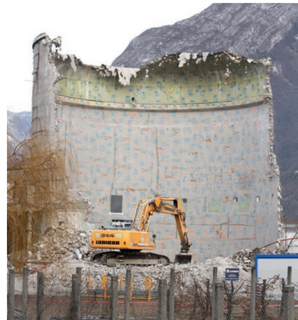
Dismantling the Siloé reactor at CEA-Grenoble.
